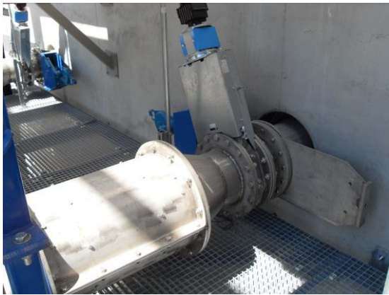
Screw press with safety slide valve
