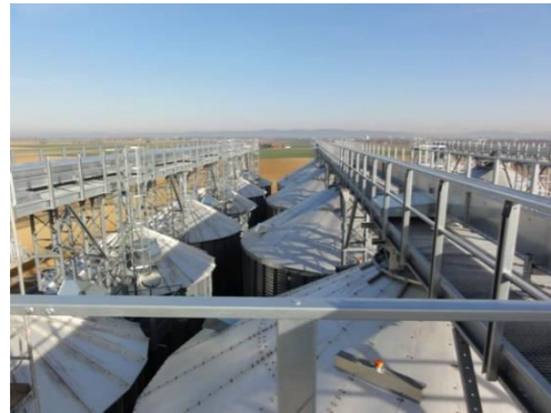
Silo runway width 2m and 2,5m
