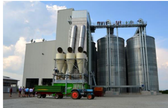
View drying plant and silo
