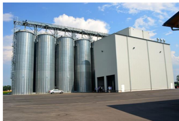
Input hall and silos
